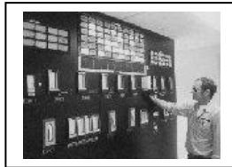
1970's Water Treatment Computer
