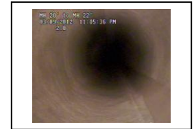
21 st Century Pipe Lining
