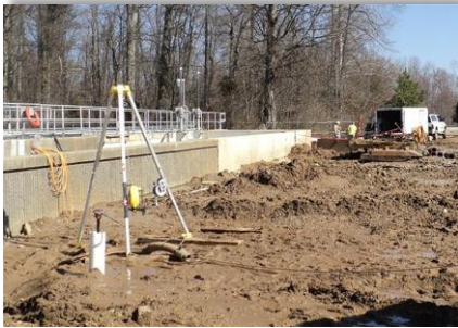
Treatment Plant Construction
