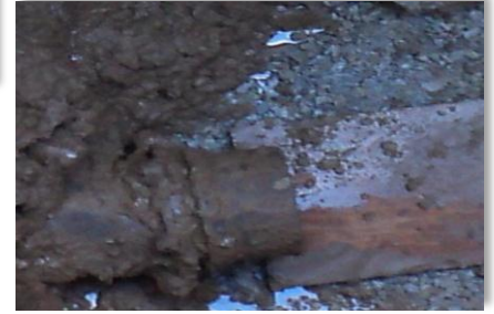
Entrance to Existing Steel Pipe
