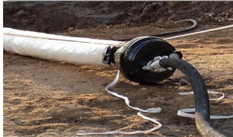
Flow-Liner® Being Steamed Cured
