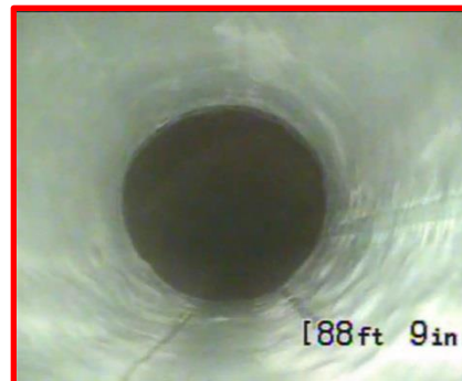
10” storm pipe after Flow-Liner® Installation
