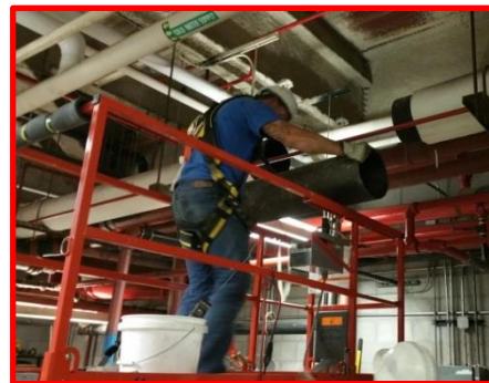
Section of 10” pipe removed for access point to install liner
