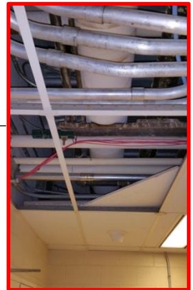
10” storm pipe after Flow-Liner® Installation
