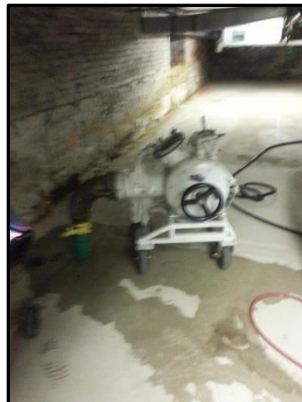
Flow-Liner® Equipment Set-up
