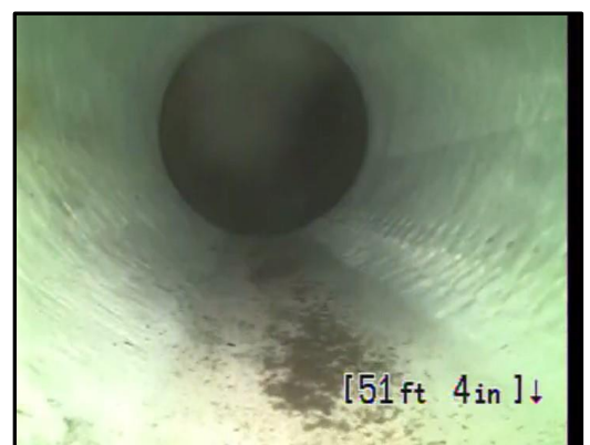
Cast Iron after Flow-Liner® installation
