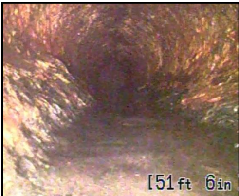
Cast iron before cleaning and lining
