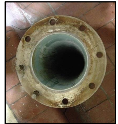
Process Piping after Flow-Liner® installation
