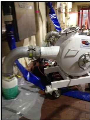
Flow-Liner® Equipment Set-up
