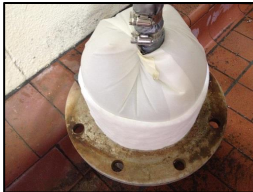
Flow-Liner® During Curing Process
