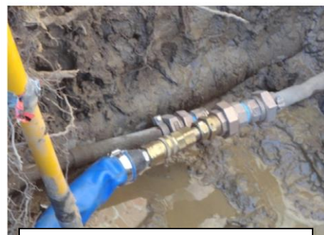
Installation of Neofit® in existing water service pipe
