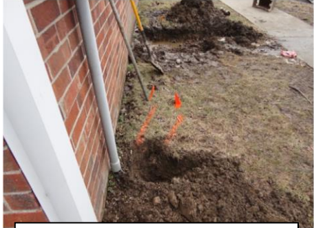
Only one minor excavation site
