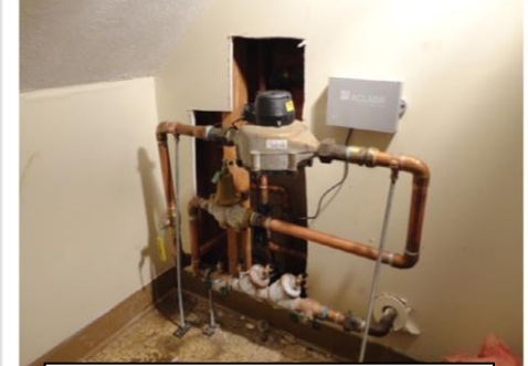
Existing access through inside wall
