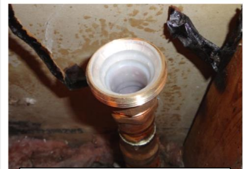
Water service pipe after Neofit® was installed
