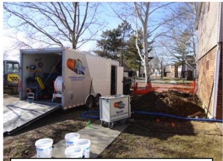
Neofit® Equipment Set-up next to building
