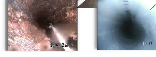
**Problem:** A newly remodeled medical office had a badly deteriorated underground cast iron sewer pipe. In some locations of the cast iron the bottom of the pipe was missing due to excessive deterioration. The pipe was also heavily scaled and had become a drainage issue prior to the medical office's grand opening. The building was previously home to the local Social Security Office for over 40+ years.
