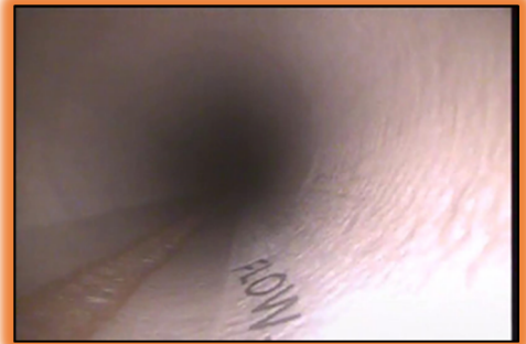
4 inch conduits after Flow-Liner® CIP Conduit Lining installed
