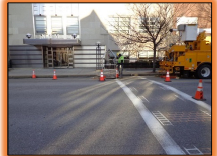
Manhole Access in the Street
