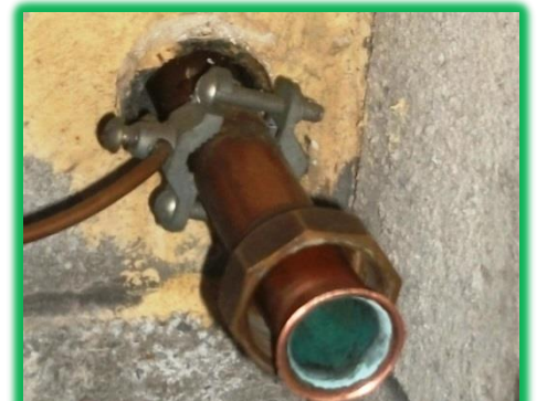
Water service line after Neofit™ installed
